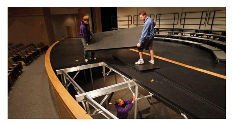
The Wenger Corporation Orchestra Pit Filler is a strong yet open column-beam system that's simple, fast and flexible to set-up or take down and features solid acoustically dampened decks with independent adjustment for a seamless fit.
